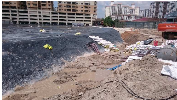
Figure 3: MVC for ground improvement works
