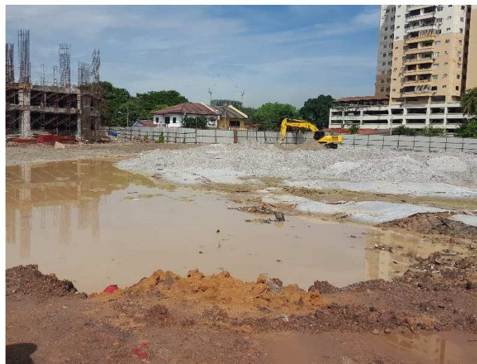
Figure 1: Site preparation for ground improvement works
