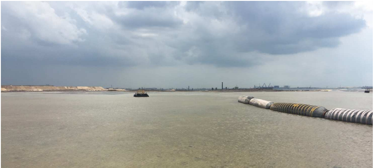
Figure 1: View of the Vacuum Pit Under Filling
