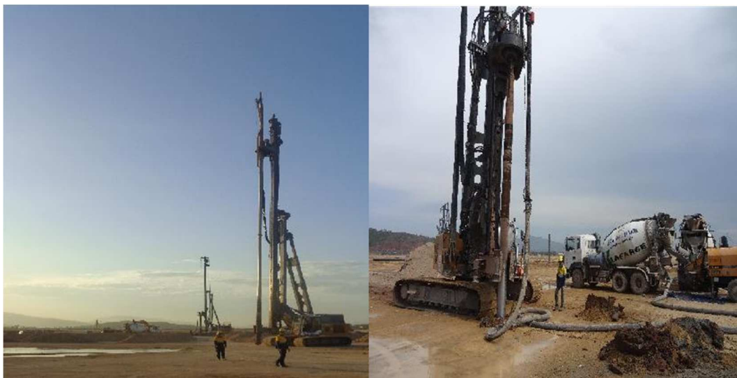
Figure 2- Menard CMC rigs' operation on site
