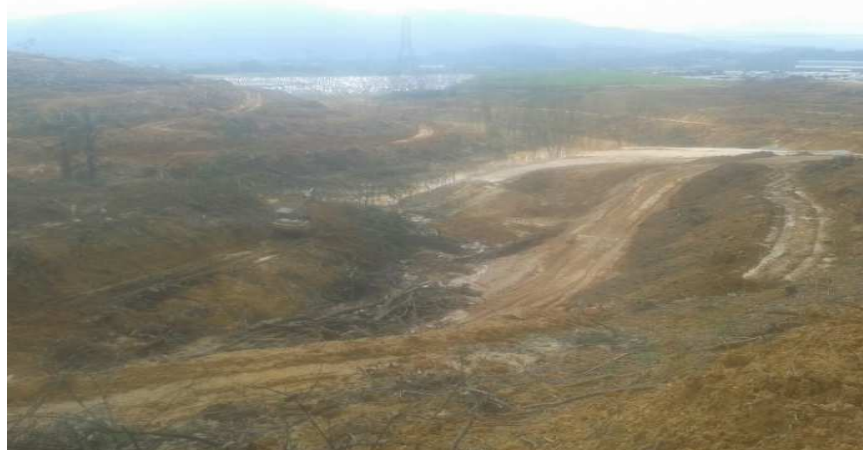
Figure 1: Site clearance for ground improvement works
