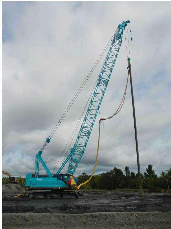
Figure 2: Stone Column Equipment at the Project Area
