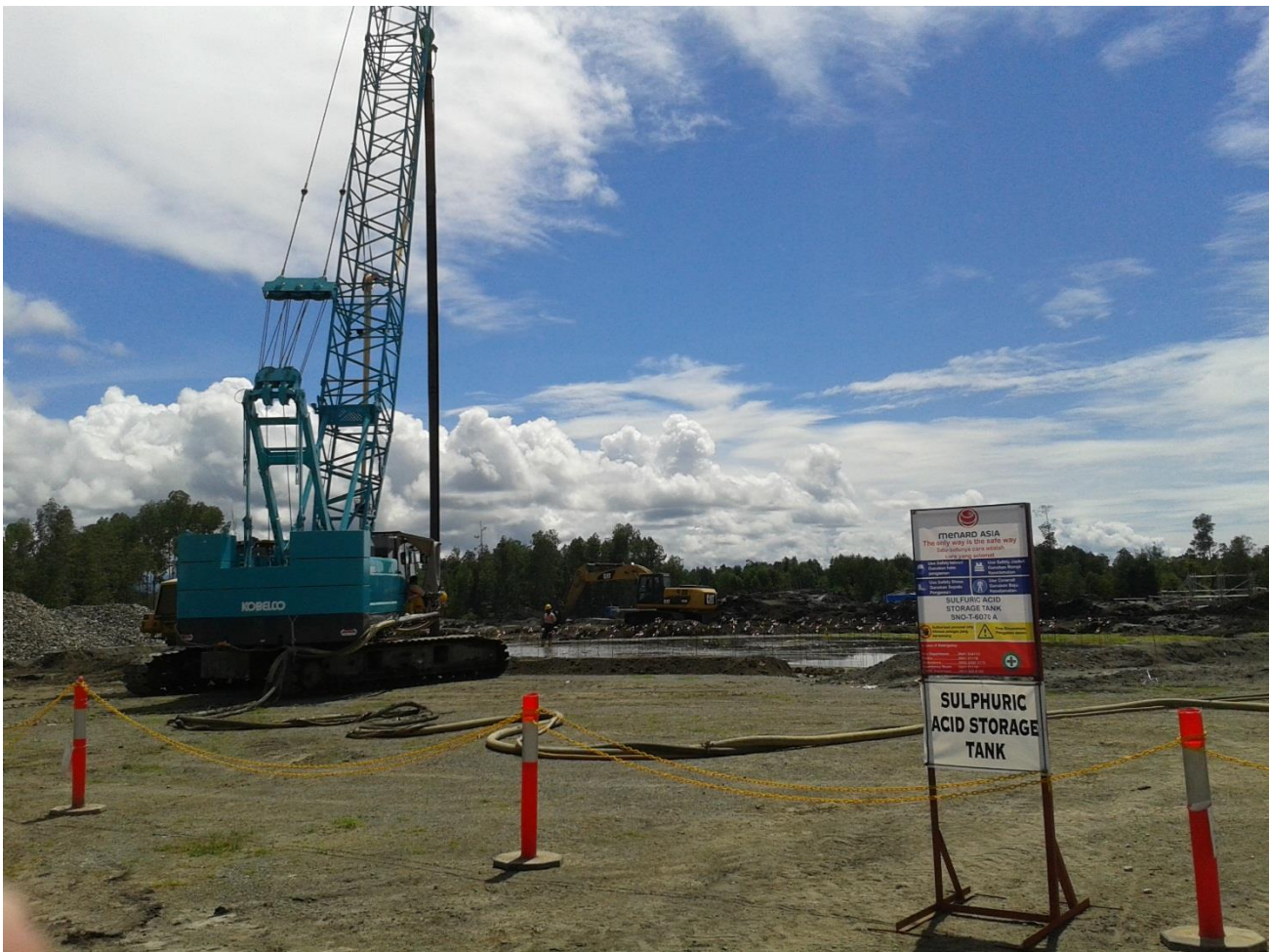
Figure 1: View of Senoro Gas Development Project Area– Soil Improvement Works
