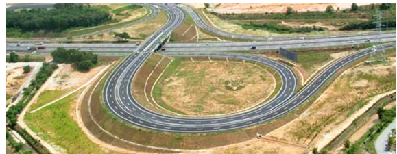
Bukit Gambir interchange open to traffic
