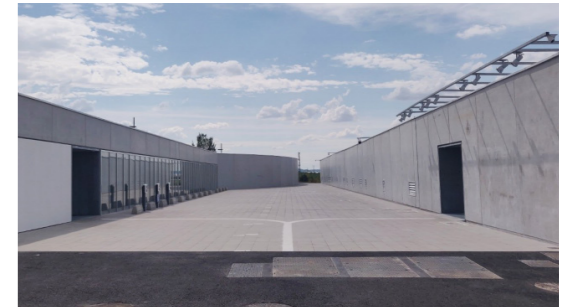
Data Center in Peltre (France)
