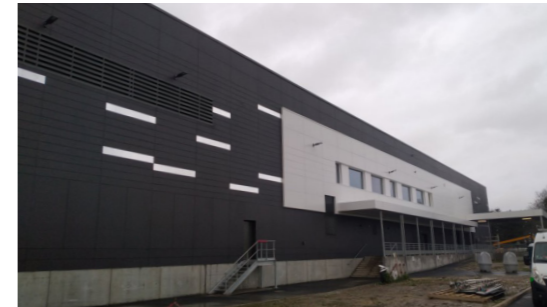
Verlinghem Banking Data Center Project (France)
