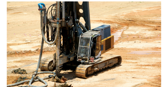
Nghi Son Refinery (Vietnam)
